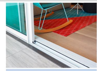
Threshold drainage is an ideal solution for protection against water from the outside while still providing a continuous accessible path between the inside and outside.
